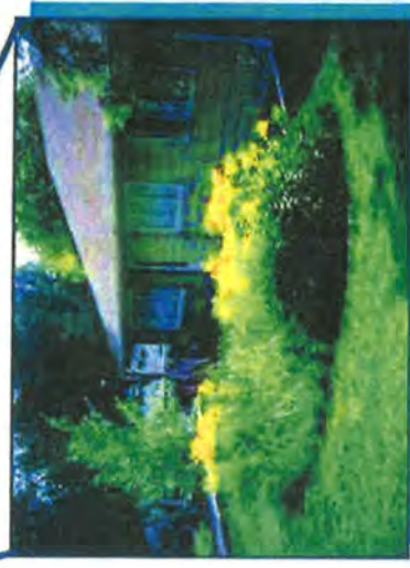
Rain Gardens are shallow depressions planted with native plants and are positioned to capture stormwater runoff.
